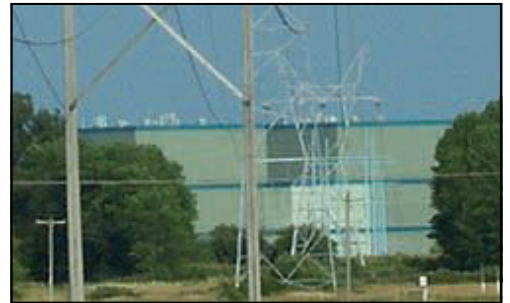
Point Beach Nuclear Power Plant
